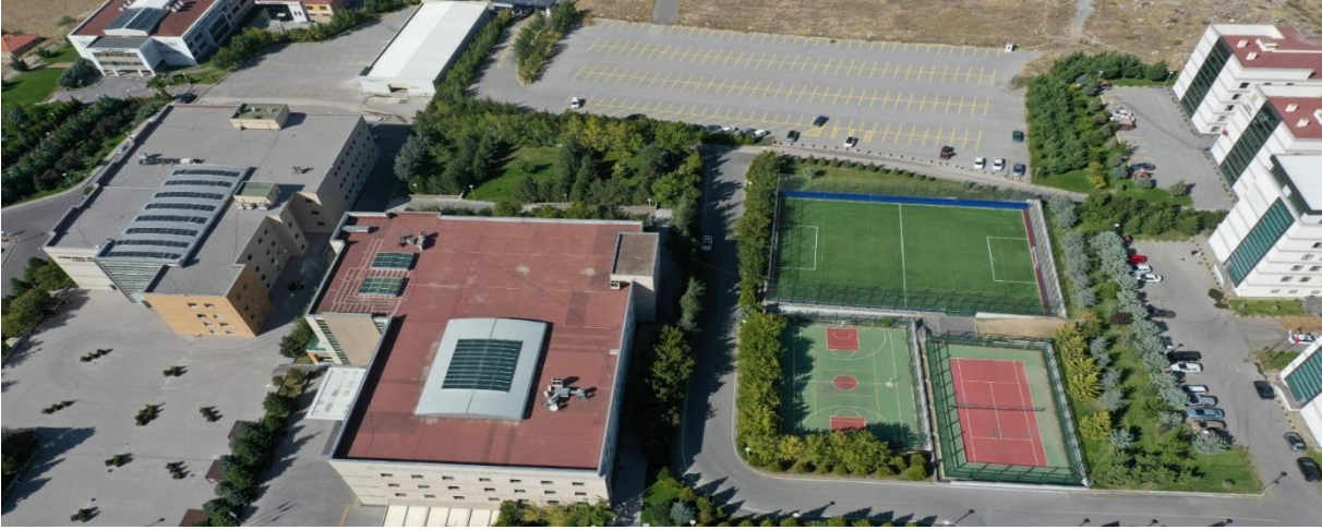
Image: Central Campus Rectorate and Faculty of Applied Sciences Roof Natural Lighting View
