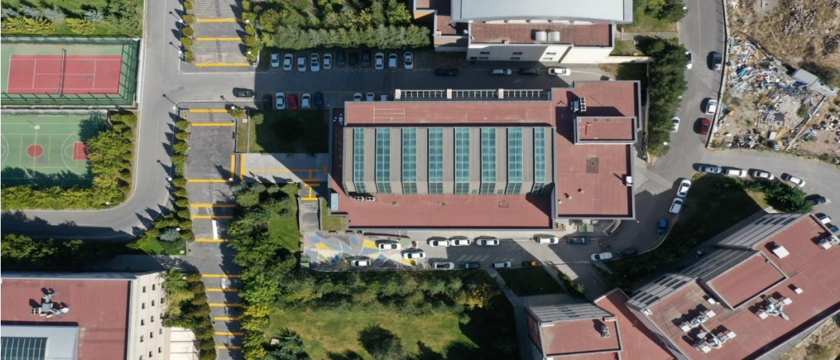
Image: Central Campus Technical Sciences Vocational School Roof Natural Lighting View
